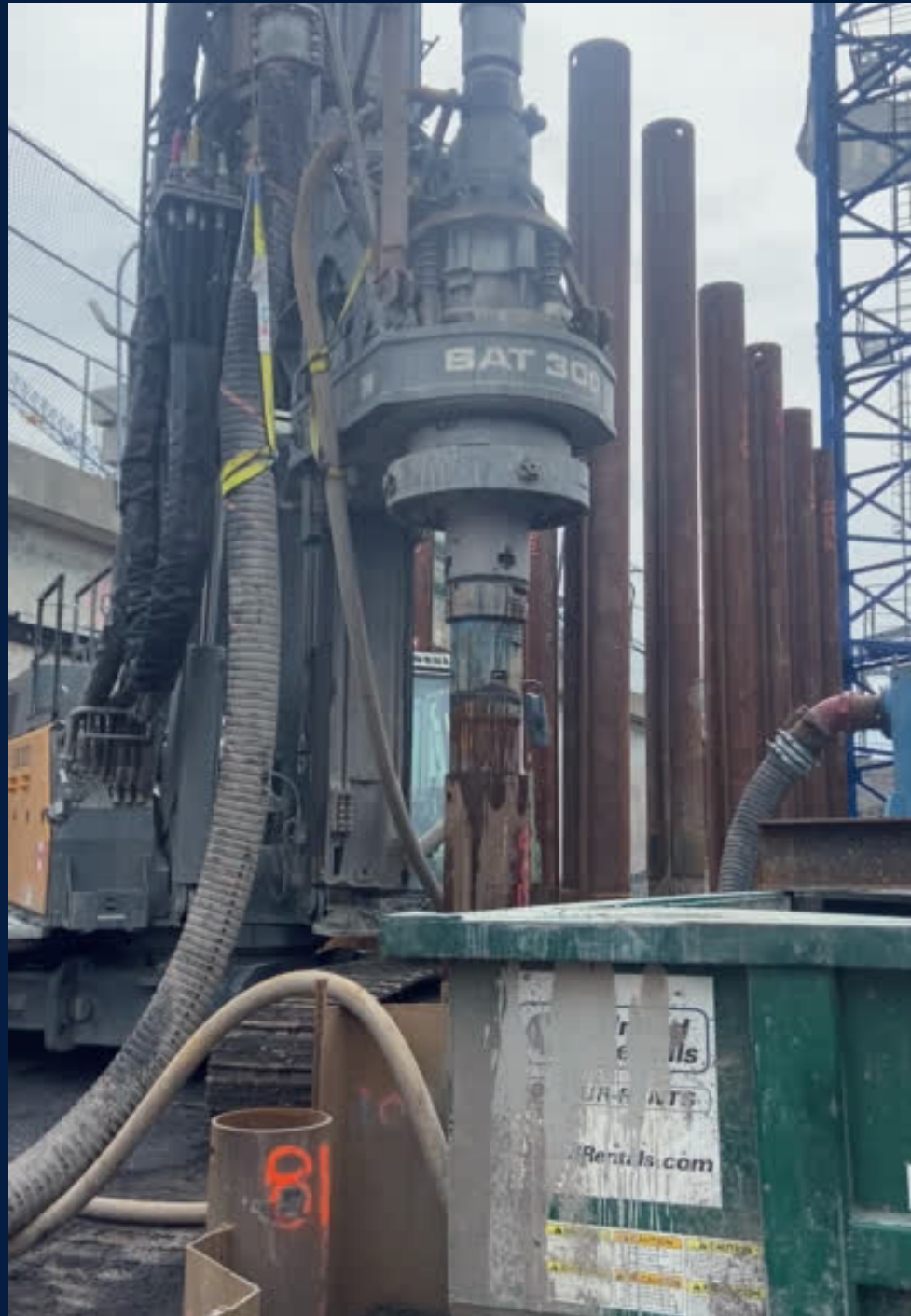
LB 30 drilling 16" piles with casing advancement system for combi wall
